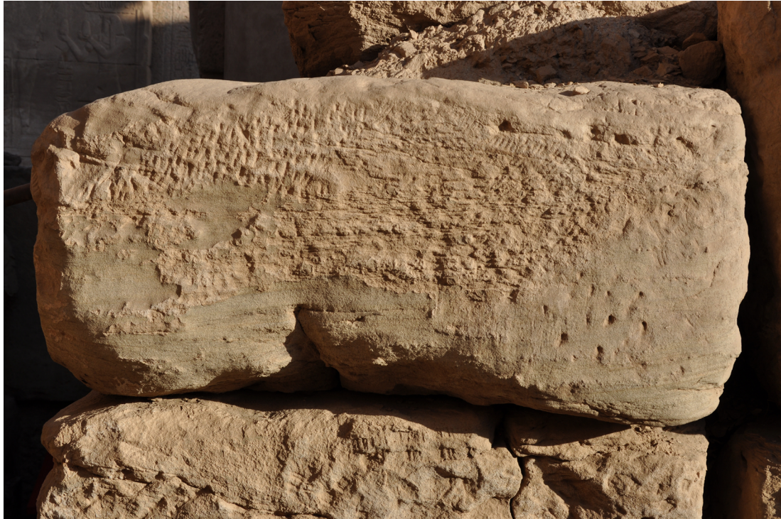
Fig. 8. Greenish sandstone block in the 5 th pylon at Karnak temple. Note the chisel marks.
